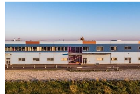
Metal Industrial Facility
